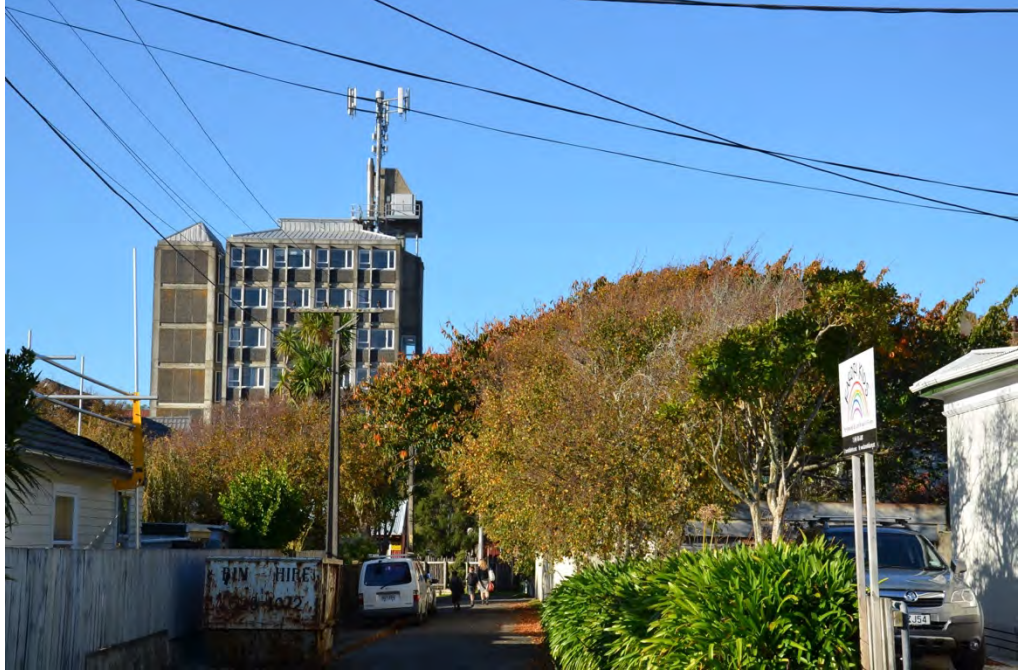
Figure 11: A view from Campbell Street, looking eastwards along the lane leading to the 'Karori Kids' pre-school and play-centre. The 10 level Malcolm Block with the telecommunications aerials attached to its roof is clearly visible on the skyline.
