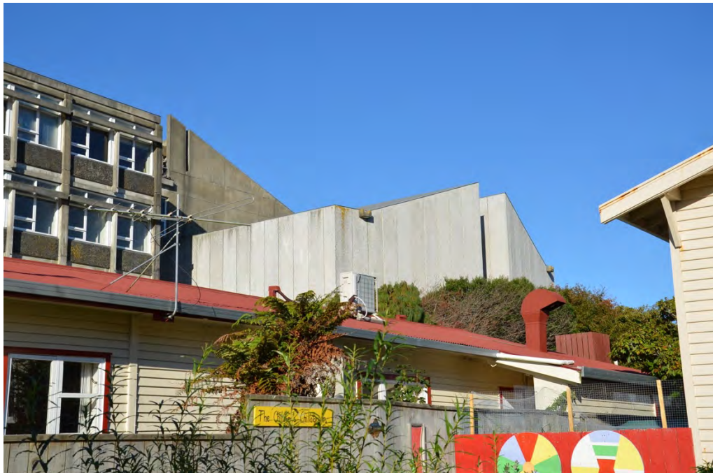
Figure 10: The former 4 storey Panckhurst Block (left) and the 3 storey Drama Theatre 'Block' (right) on the Site, to the east of the red roofed, single storey Oke Pai Marae building (also on the Site) and the corner of the 'Karori Kids' pre-school and play-centre on the extreme right of the image.
