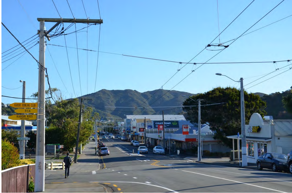
Figure 40: The view of the Karori Shopping Centre, looking westwards from just east of its intersection with Campbell Street.
