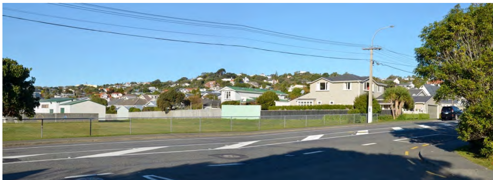
Figure 16: The residential properties at 45 and 49 Campbell Street at the western end of the southern boundary.
