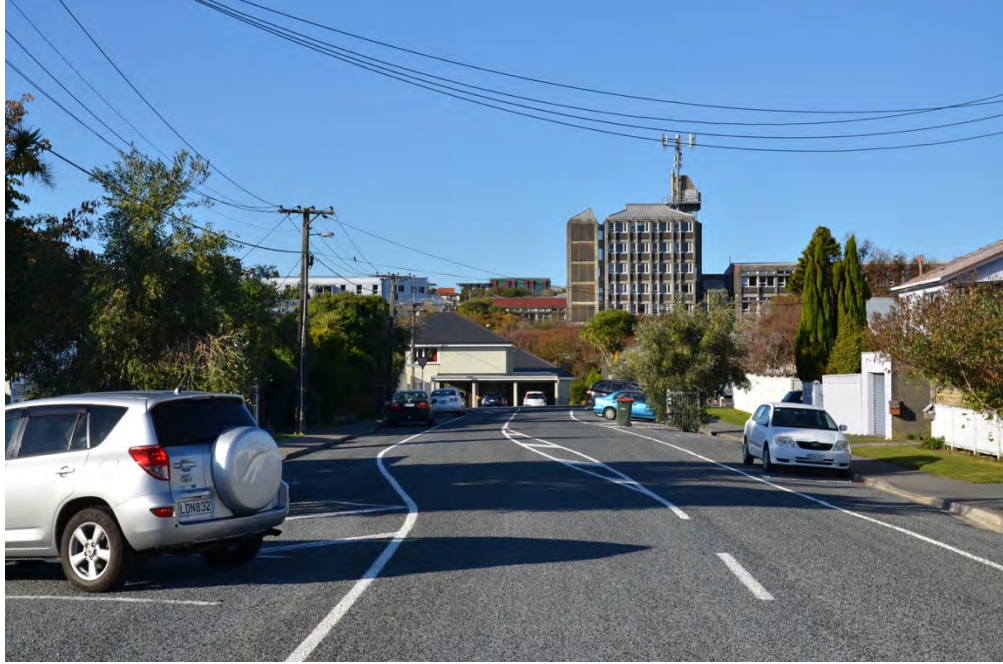
Figure 37: A view of the Site when looking east along Lower Street. The tall building with the telecommunications aerials on its roof is the 10 storey high Malcolm building which has now been demolished. To its right is the 4 storey Panckhurst Block which has also been removed.
