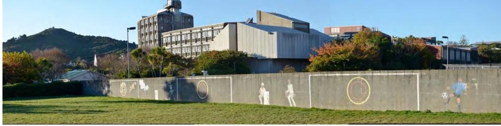
Figure 20: The view from near the Campbell Road Site boundary, across the grassed playing field, and deep into the Site. (Photograph shows buildings now removed).
