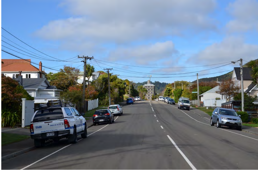
Figure 42: The highly axial and focussed view of the former 10 storey high Malcolm Block, as seen when looking southwards along Reading Street.
