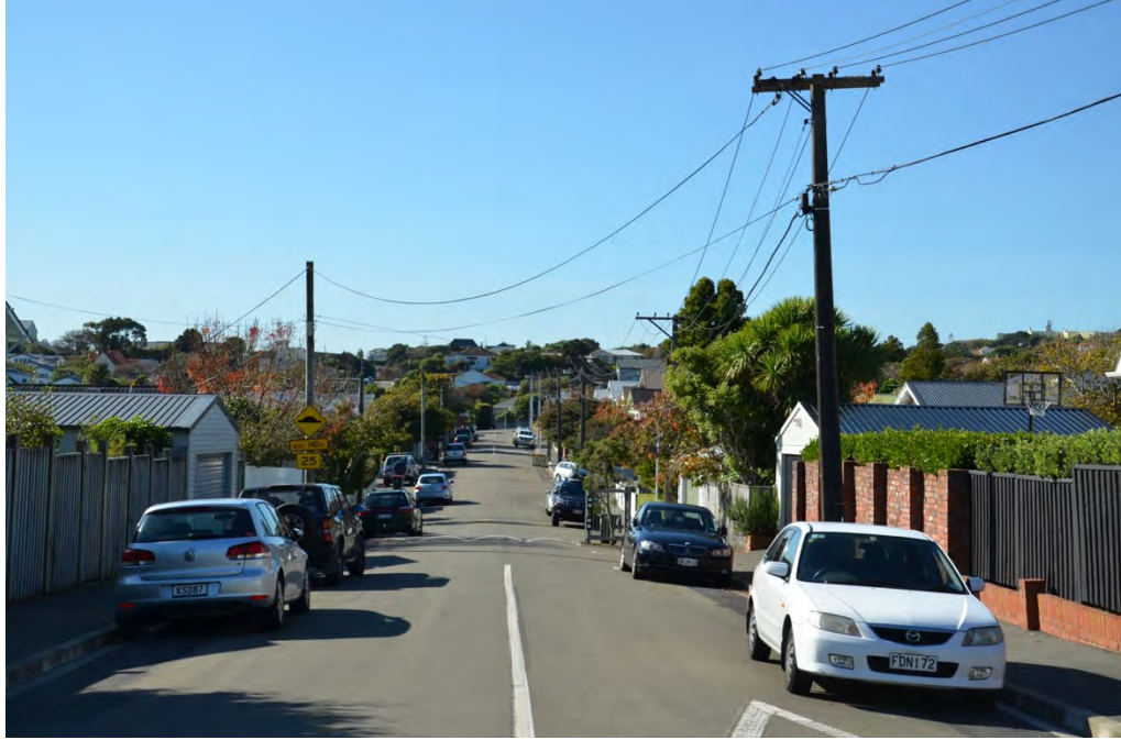
Figure 33: A view, looking eastwards, along Scapa Terrace. The properties on the left back onto the Site.
