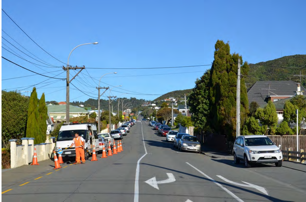
Figure 29: The view southwards along Campbell Street from its intersection with Karori Road.
