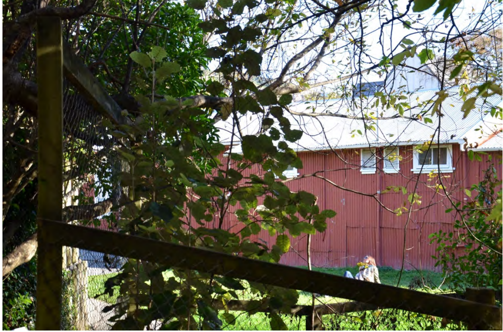
Figure 9: The eastern side of the RSA hall to the right of the base of the sloping pathway between Donald and Campbell Streets.
