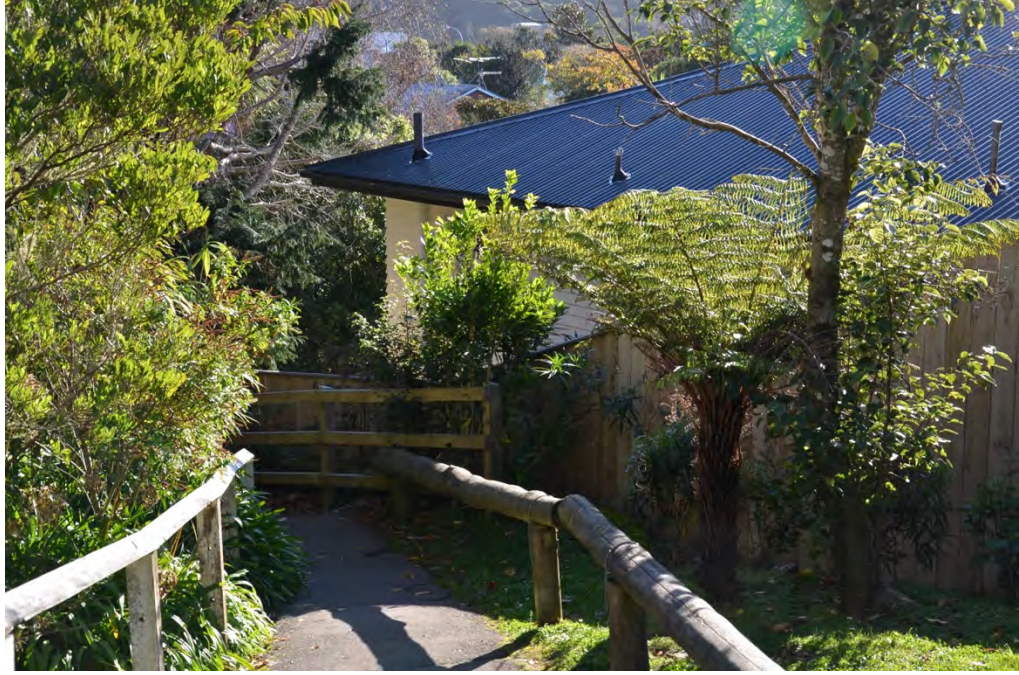
Figure 7: Looking west down the sloping pathway between the Site (on the left) and the corner of the residential property at 221A Karori Road.
