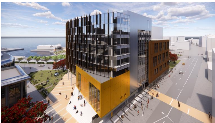
Fig 12: View of the south-western corner of the development
