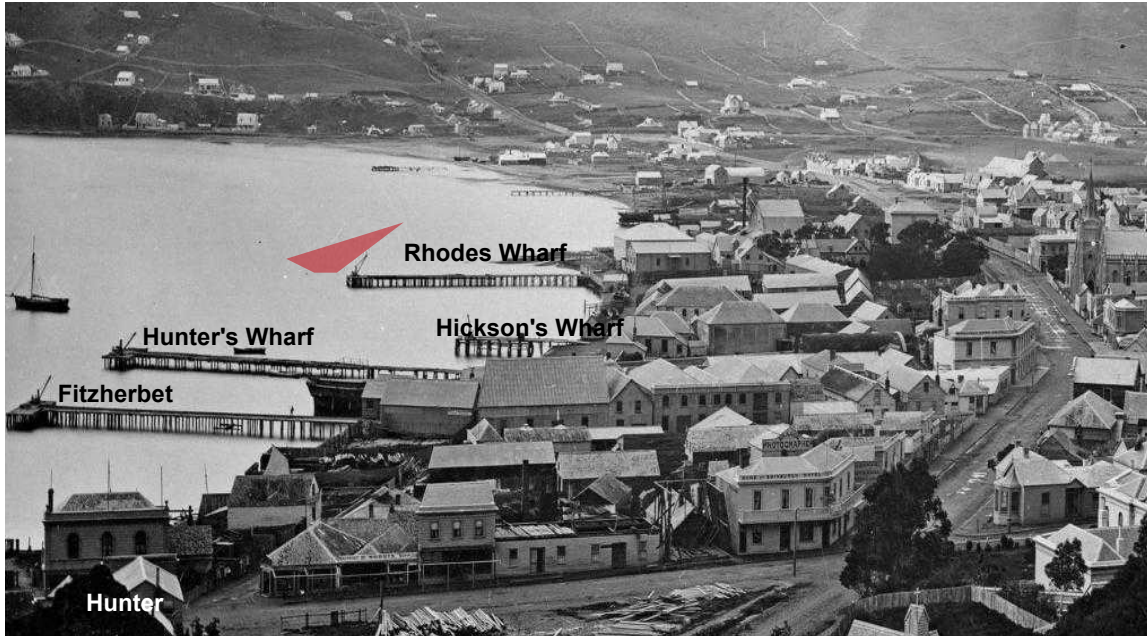
Illustration 7: Detail of Te Aro, 1869 (ATL 1/4-019551-F). Approximate location of Michael Fowler centre carpark shown in red.
