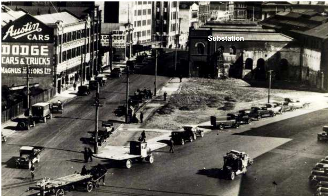
Illustration 24: Detail of corner of Jervois Quay and Wakefield Street before December 1930. Following demolition of Tramways Power House (Wellington City Libraries 50002-3-55)
