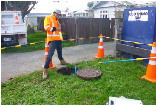
Miramar Stream manhole on grassed berm
