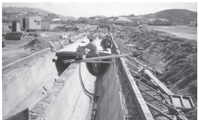
Construction of drainage channels, Wellington airport, 1957. WCC Archives 00158-2-88
