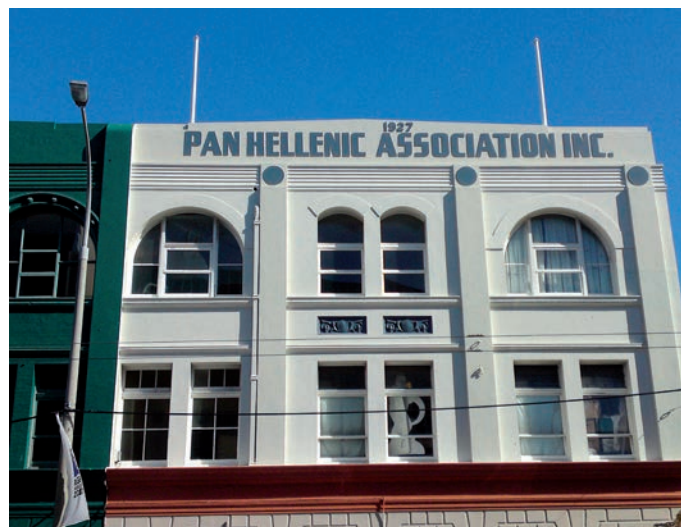
Pan-Hellenic Association building, Wakefield Street. WCC Heritage
