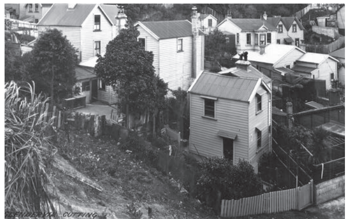
Glenbervie cutting, western access, 1929 WCC Archives 00127-0-1
