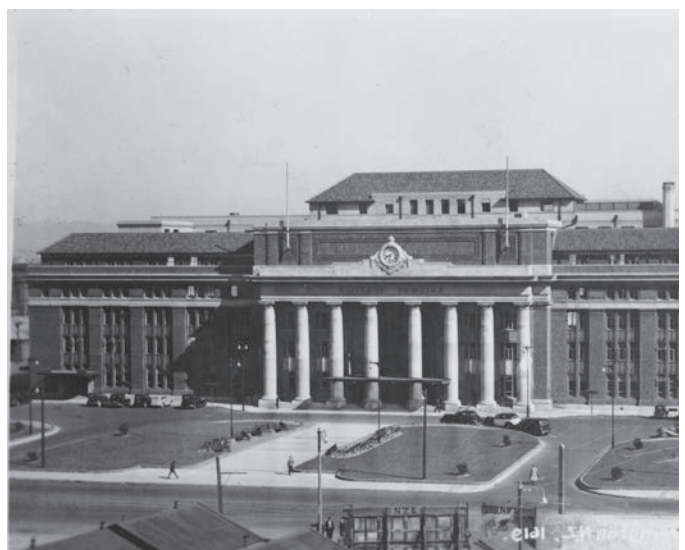
Elevated view of the Wellington railway station, Bunny Street frontage, 1930s [1937?]. WCC Archives 00138-0-865-
