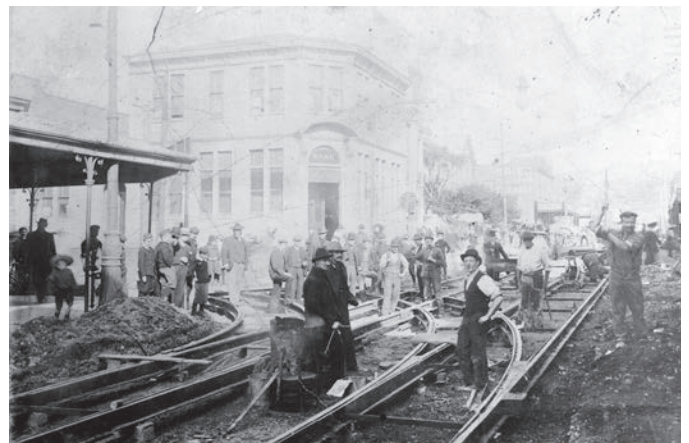
Workmen laying tram tracks corner of Vivian and Cuba streets, 1904. WCC Archives 00138-0-3187
